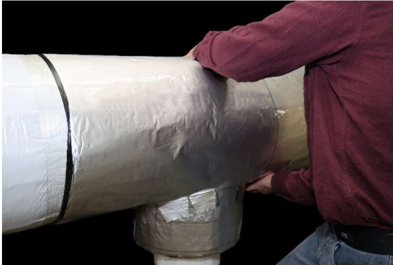
Figure 26: Main piping primary vapor barrier (Note cutouts in main pipe).
