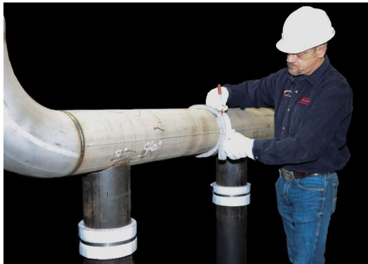
Figure 12: Cut length determination using a piece of CRYO Super Mat.
