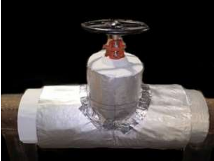
Figure 51: Vapor stop terminating below packing gland.
