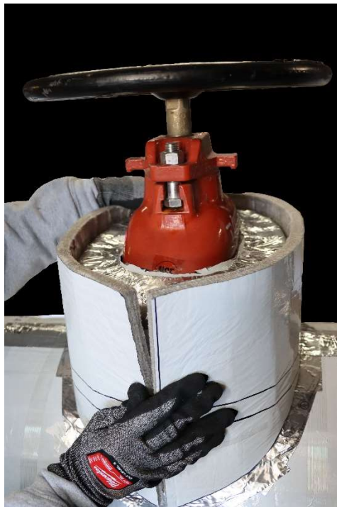
Figure 47: Final layer of CRYO Super Mat insulation.
