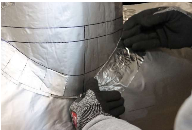
Figure 48: Installing and sealing of primary vapor barrier.
