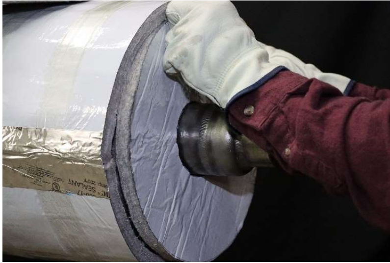
Figure 33: Successive layer of end cap installation.
