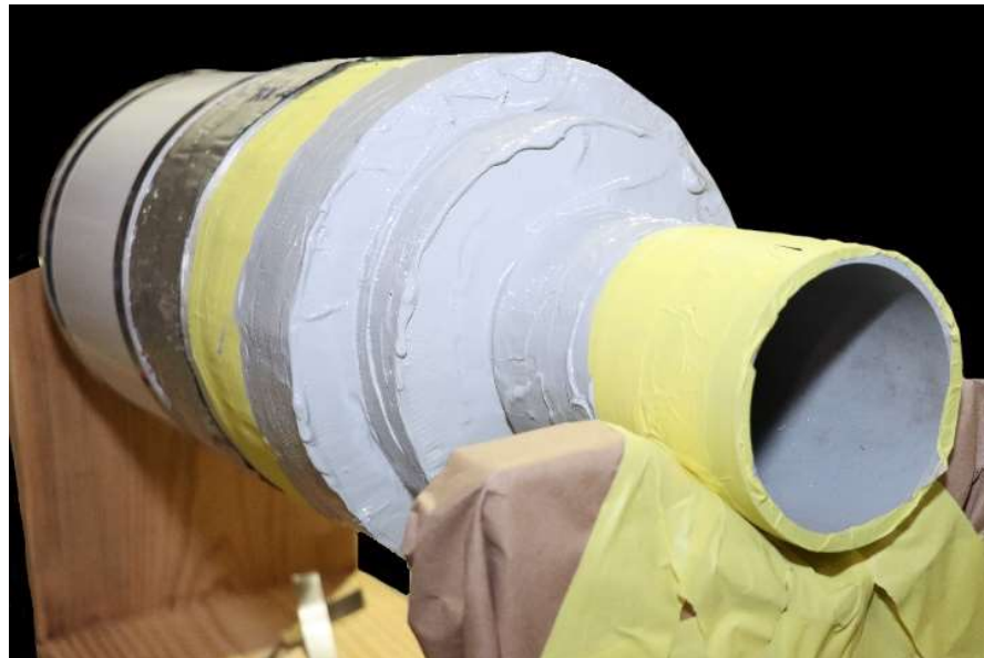
Figure 9: Second coat of mastic. Yellow tape providing for clean edge termination of mastic.
