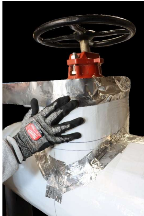
Figure 46: Butyl-based aluminum tape over secondary vapor barrier.
