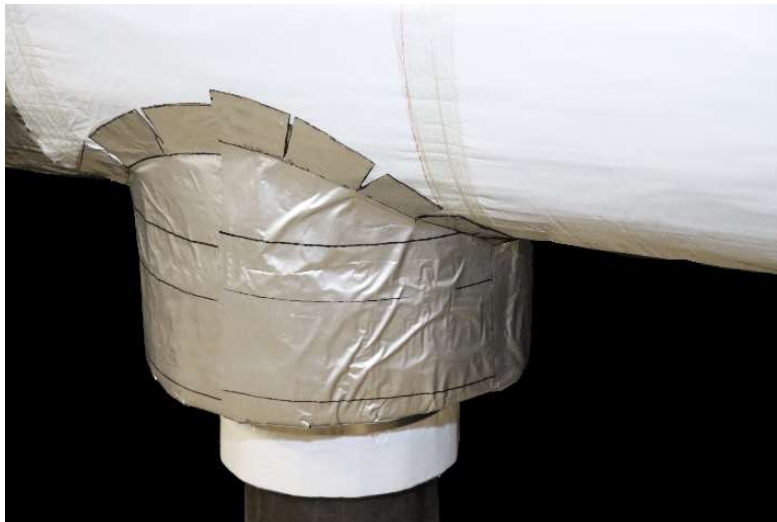
Figure 25: Primary vapor barrier over tee.
