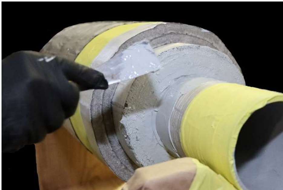
Figure 7: First coat of vapor stop mastic. Masking tape (yellow) was used to achieve clean termination of the mastic layers.
