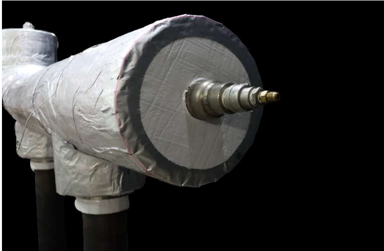
Figure 37: Use of primary vapor barrier membrane to seal tabs of butyl-based aluminum tape.
