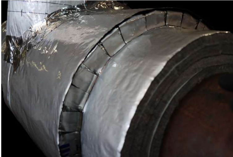
Figure 49: Sealed primary vapor barrier.
