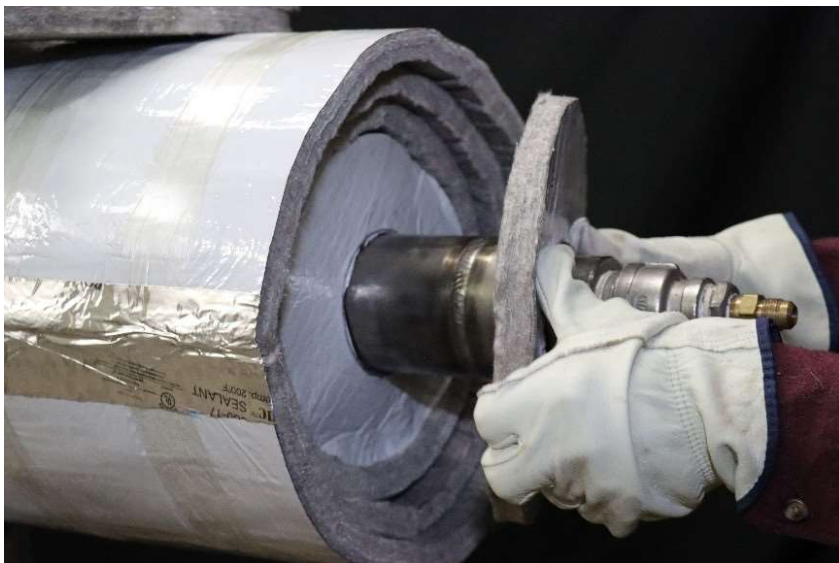
Figure 32: Successive end cap installation.
