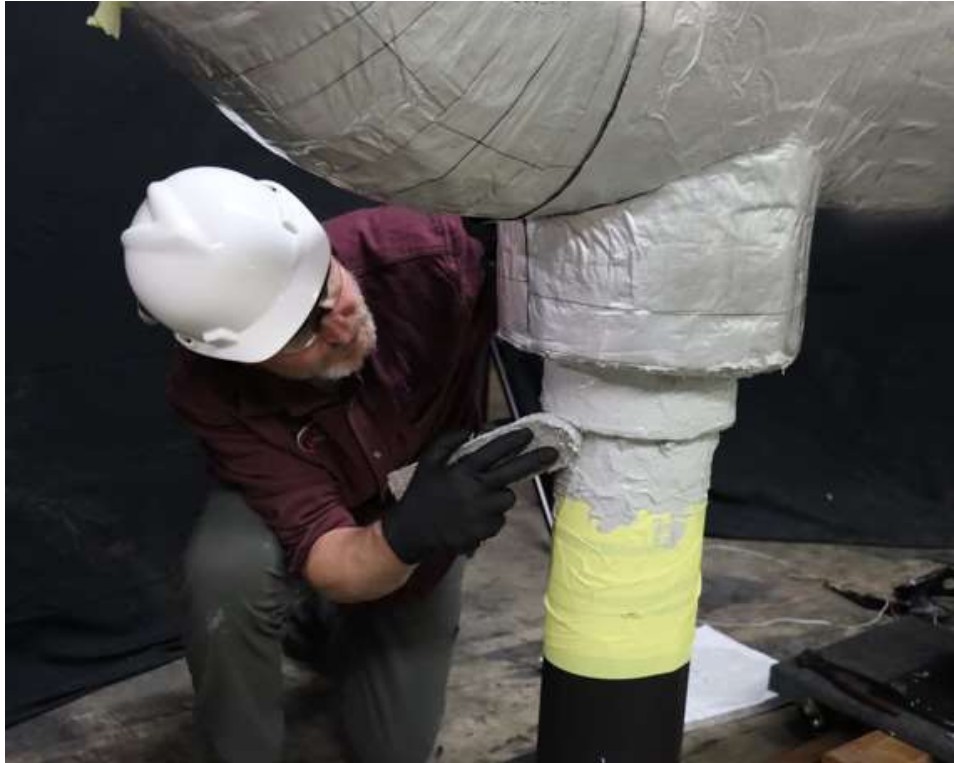
Figure 28: Example of continuous mastic type vapor stop over termination of tee.
