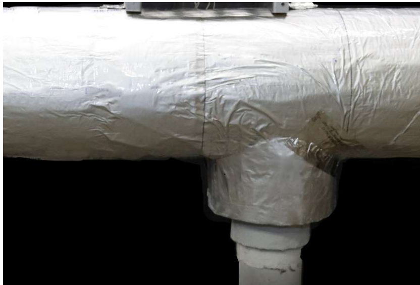
Figure 27: Primary vapor barrier joint sealed with either butyl-based aluminum tape or a strip of vapor barrier membrane.
