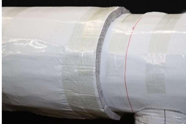
Figure 15: Second layer with offsetting joints.
