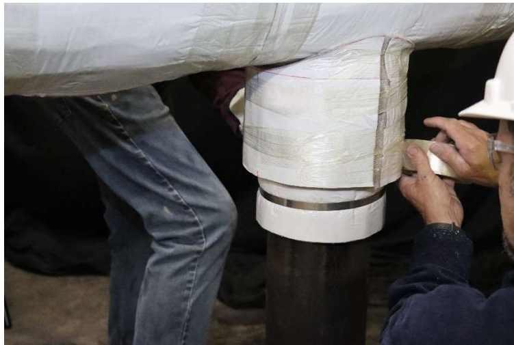
Figure 23: Dummy leg or tee insulation piece secured using glass reinforced tape. Note the full, continuous contact of the branch PAP foil onto the main pipe PAP foil.
