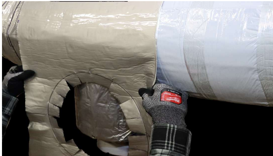
Figure 5: Installing primary vapor barrier.
