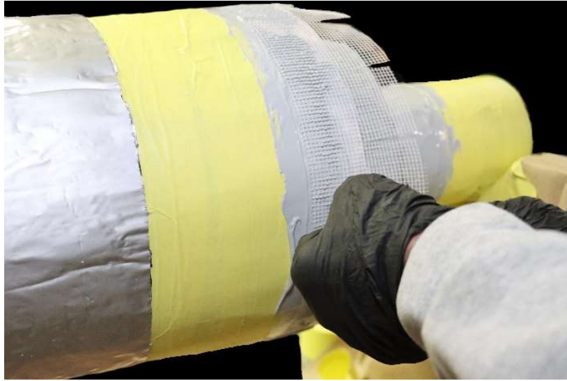
Figure 8: Imbedding reinforcing membrane into the first coat of mastic. Masking tape (yellow) was used to achieve clean termination of the mastic layers.
