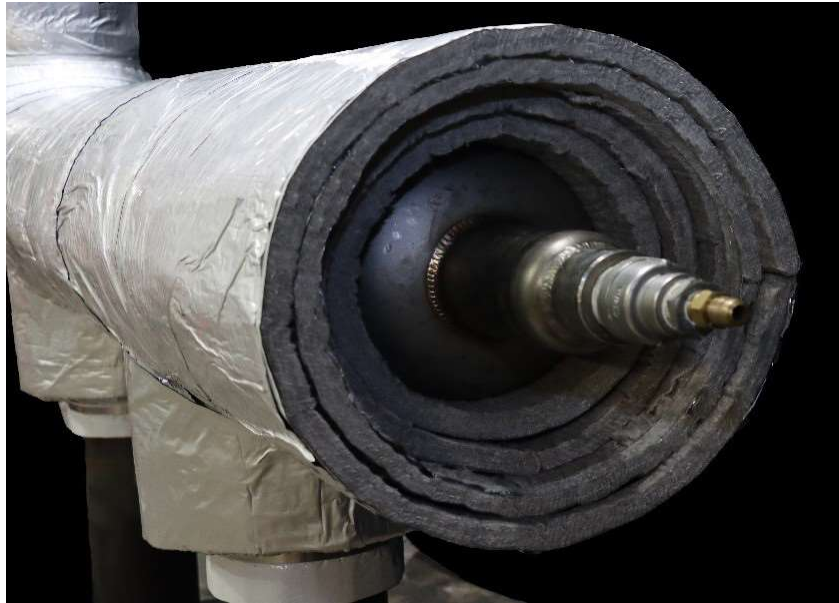
Figure 29: Pipe insulation termination at the pipe end cap.
