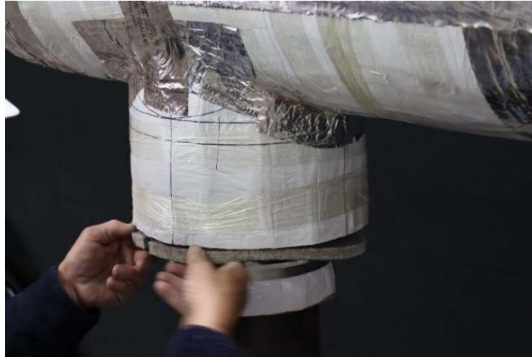
Figure 24: Photo depiction of butyl tape to achieve a secondary vapor barrier layer and an installation of an insulation disk to achieve a stepped construction.
