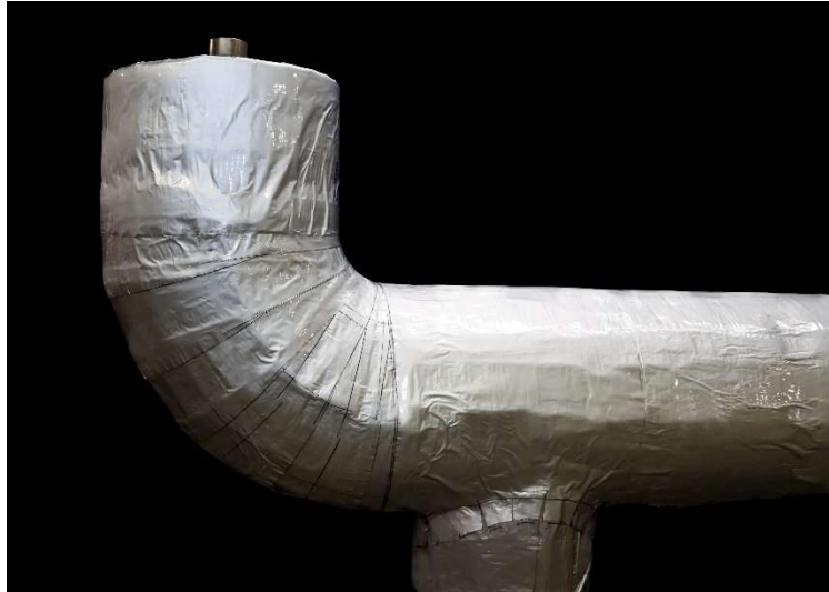
Figure 21: Primary vapor barrier membrane sealing outermost layer.
