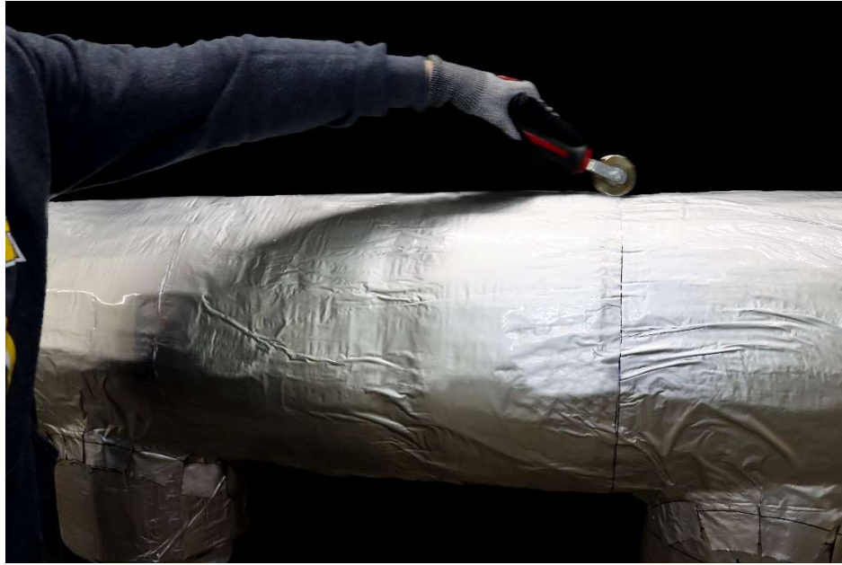
Figure 6: Use of roller to smooth out wrinkles.
