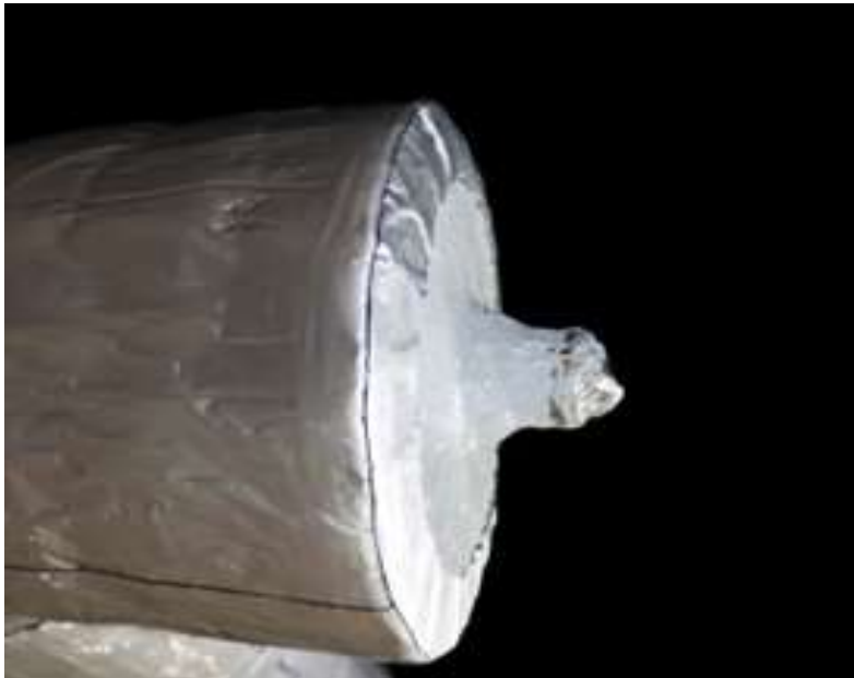
Figure 38: Vapor stop applied to the pipe nipple to overlap the primary vapor barrier.
